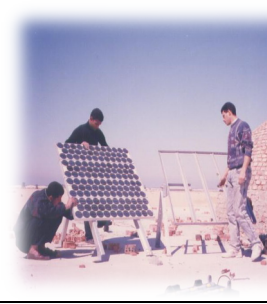
Fig. (20): The trained members are installing the house solar power units.
