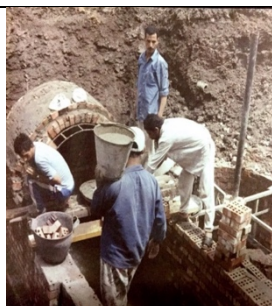
Fig. (14): Building a Biogas Plant in the Village by villagers.
